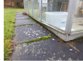
P11: Cill fixing defect
