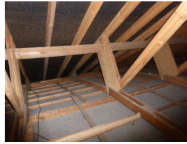
P11 & 12: Typical roof structure
