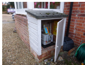
P29: Gas meter housing
