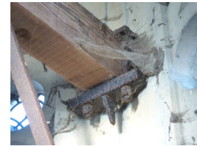
P49: Headstock beam bracket
